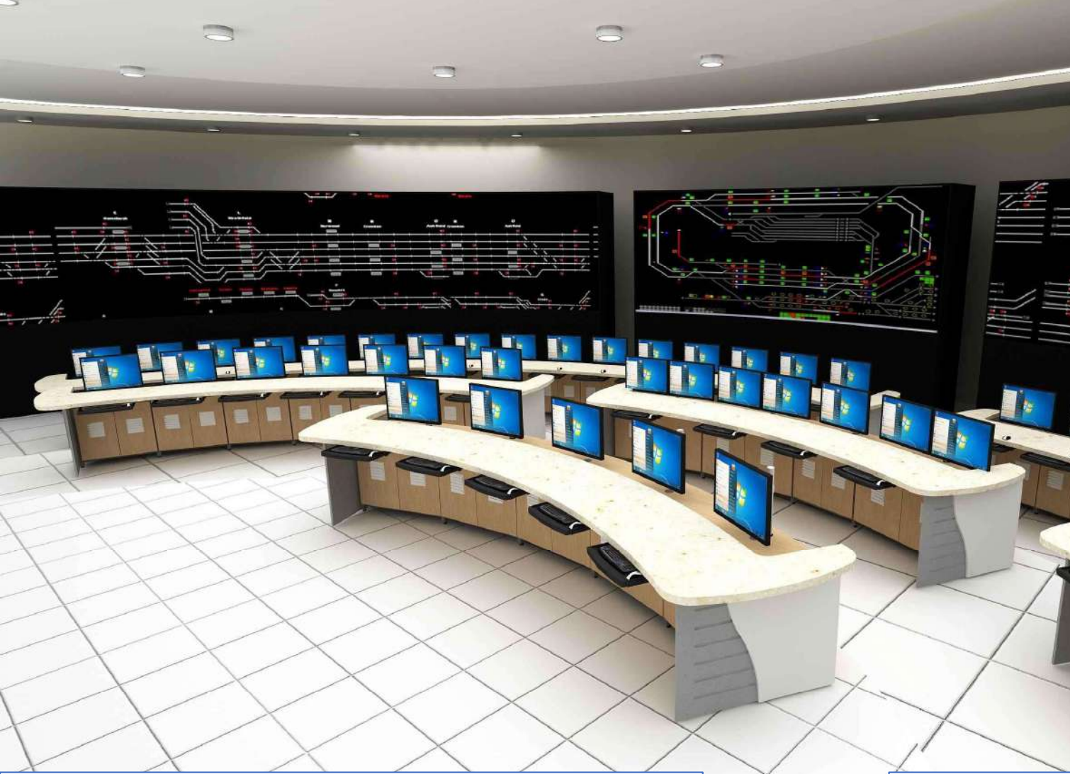
And Station control desk of Phase 1
