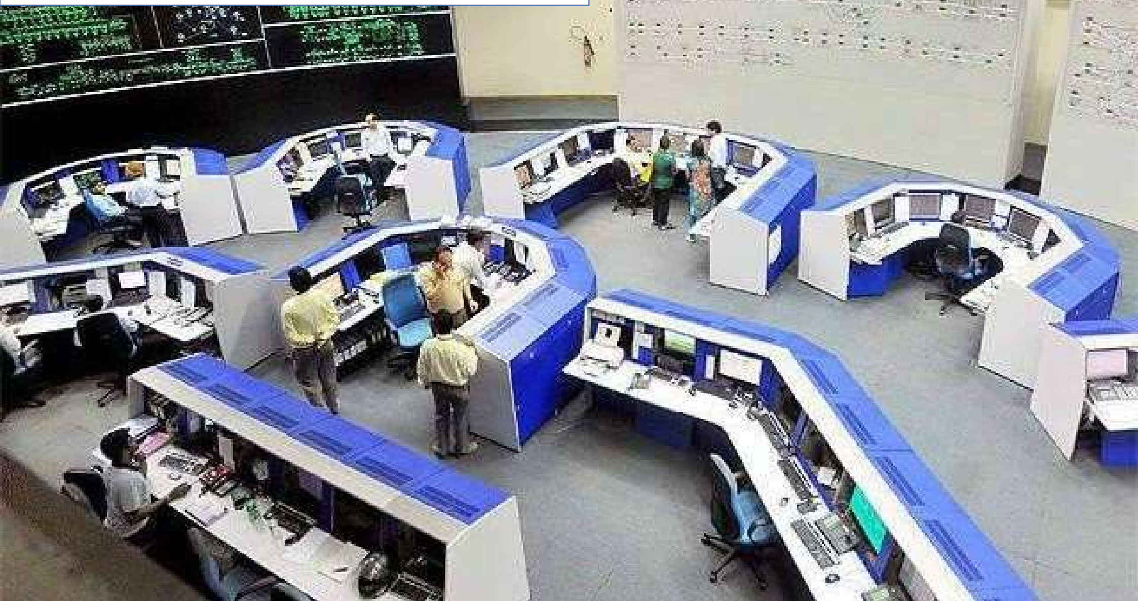
DELHI METRO SHASTRI PARK (Part of the Project )
